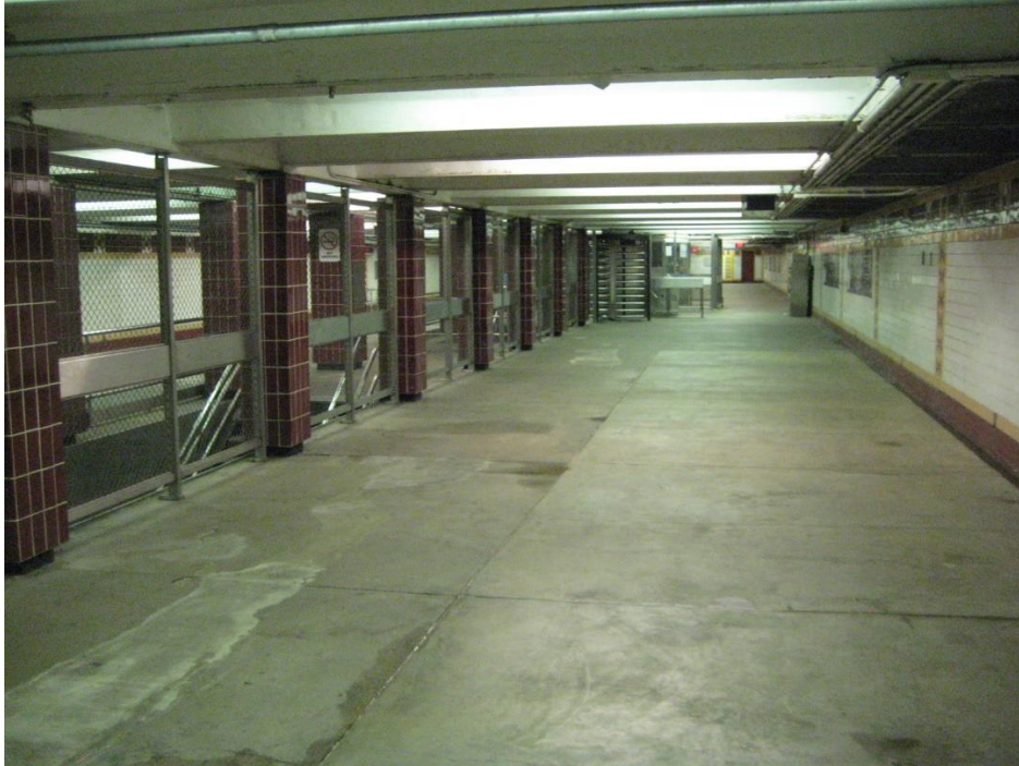
Photo 3: First underground level at Lombard and South station. Passengers have to walk all the way to the center of the first underground level to enter the tollbooth.
