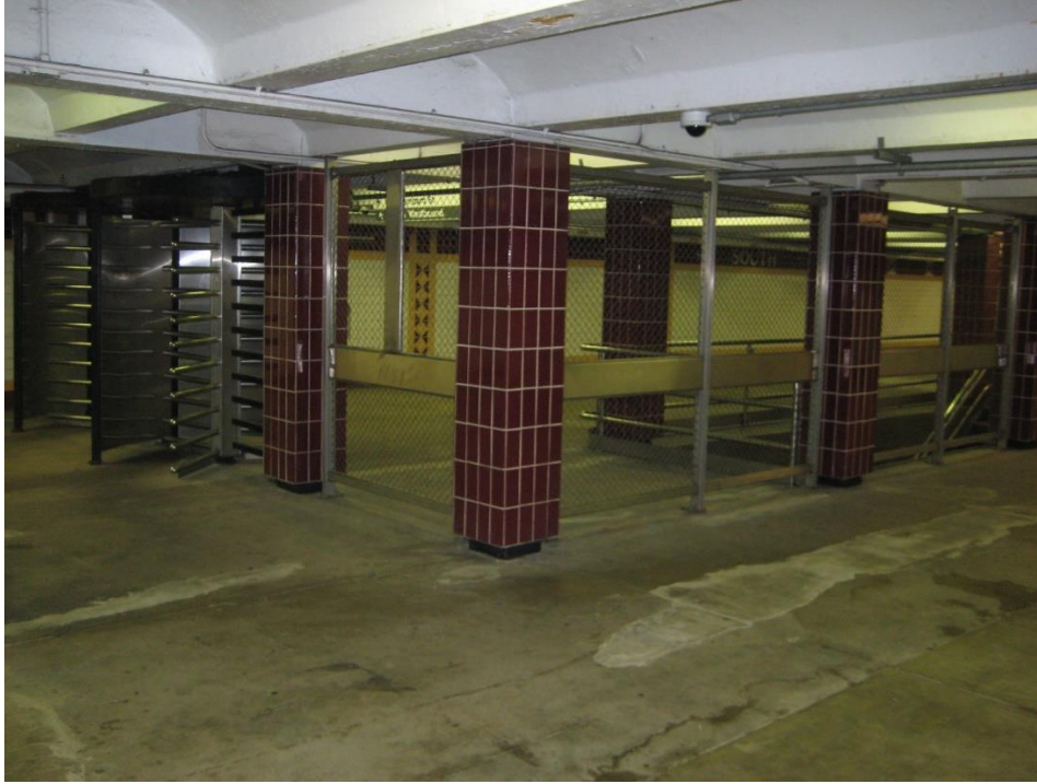
Photo 2: Exit at the first underground level at Lombard and South station. Note the stair leads to the platform but no entry to the stairs from this side.
